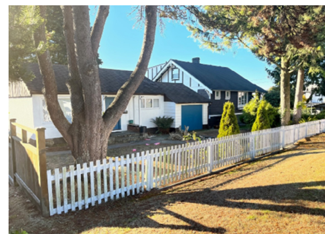
509 EAST 6TH - NORTH EAST CORNERY LOOKING AT SUBJECT PROPERTY
